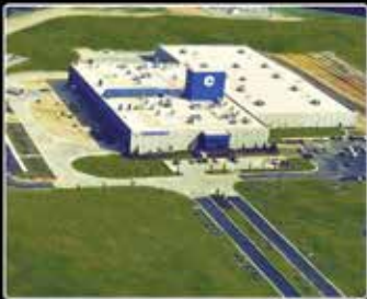
PAGELAND, SC Bronze Foundry and Manufacturing Plant
